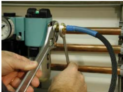
Screen 5- 6 Double Wrench technique
